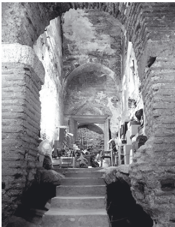
Fig. 3 Antechamber of the Large Hall, view from west. The partially demolished cross-vault of the post-sixth-century substructure and the recently built staircase in the foreground
